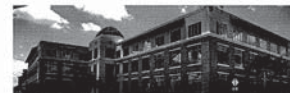
(3 story office building features architectural domes, decorative canopies, Vitrocon reflective glass, cast stone and brick veneer)
