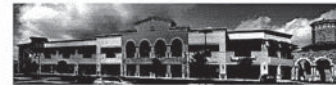
(Section of the 2 story retail center features architectural effects such as stone archways and columns to enhance the Tuscan theme)
